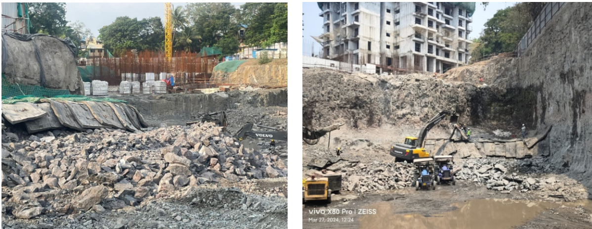
Figure.6 Two layered muffling system used to control flyrock.
