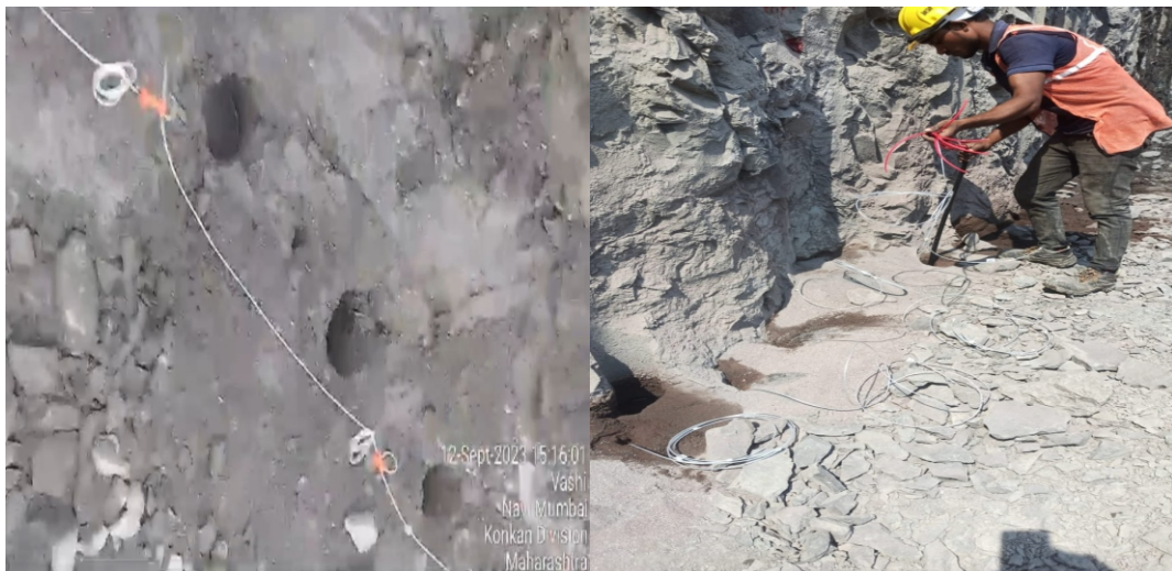
Figure 5. Pre-split blast charging with creation of crack holes
