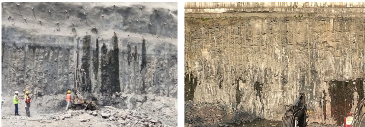
Figure 3. Line Drilling with projections of half cylindrical holes after excavation by blasting.
